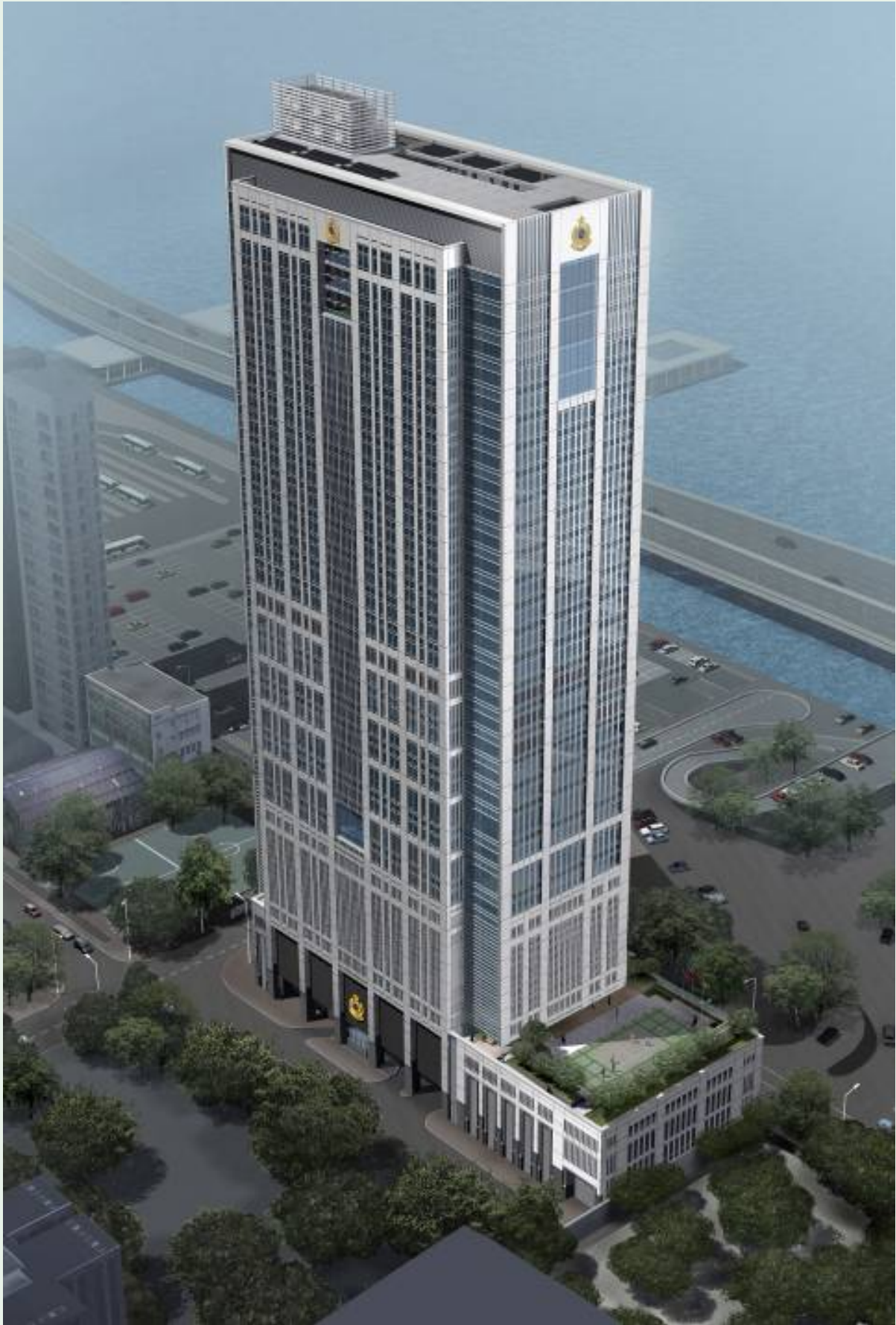
New Customs Headquarters Building – Scheduled for commission by the end of 2010
