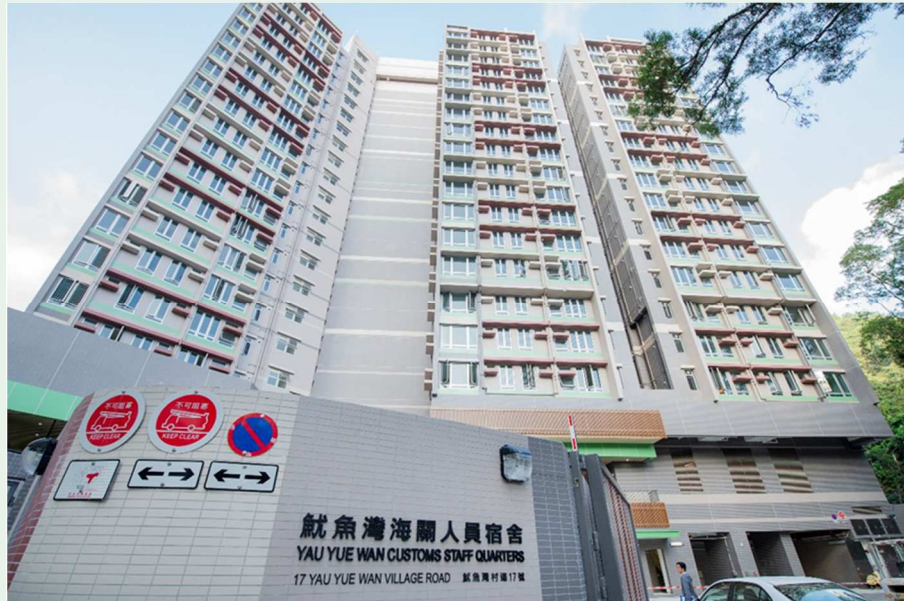
Yau Yue Wan Customs Staff Quarters provides 136 units of departmental quarters.
