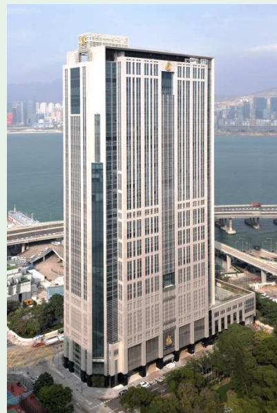
The Customs Headquarters Building in North Point
