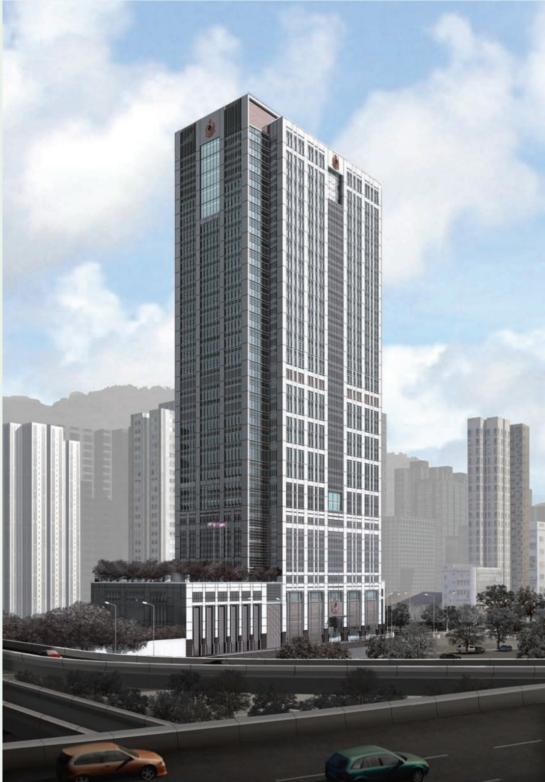
New Customs Headquarters Building – Scheduled for commission by the end of 2010
