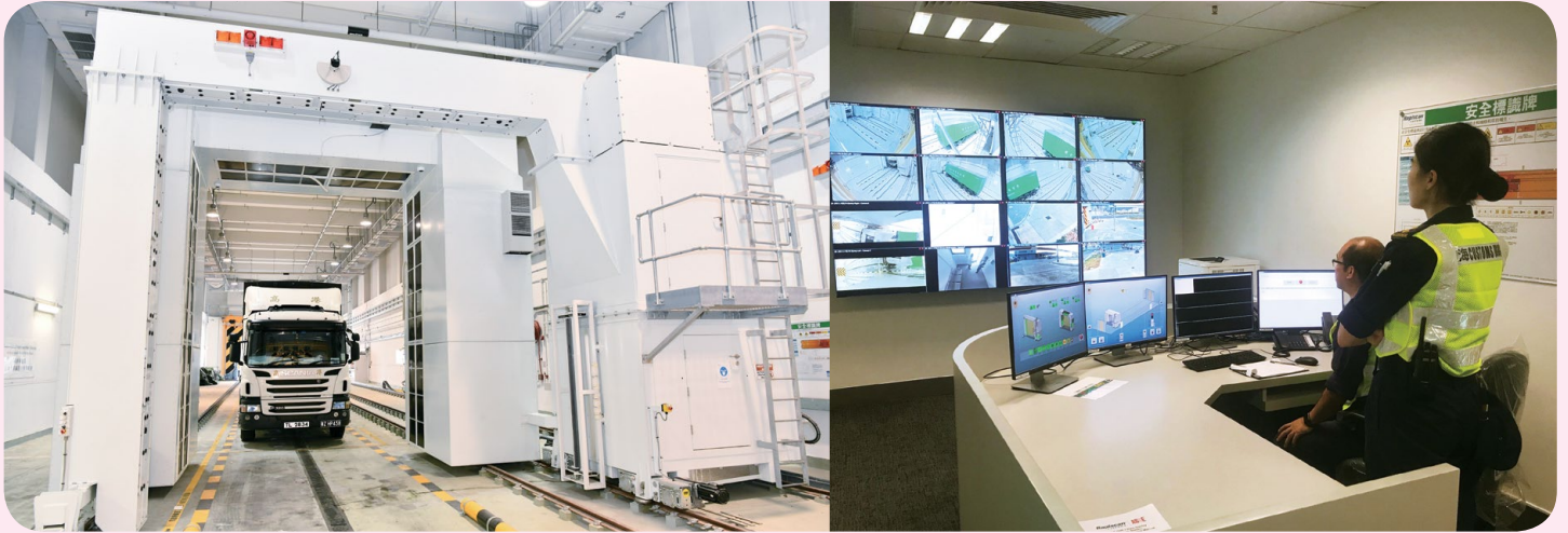
Details of goods carried by trucks are instantly revealed under the Gantry Type X-Ray Vehicle Inspection System at the HZMB's Hong Kong Port.
